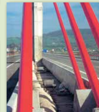
▼ PPA 571 coated suspension cable covers after ten years in Spain.
