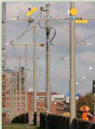
▲ These tram power pylons were coated in 1995 and twenty years later, in 2015, are free of corrosion and still look new.
